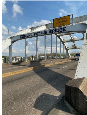
Mr. Ault visited the Edmund Pettus Bridge in Selma, AL. This is where those protesting unequal voting laws were beaten on TV.
